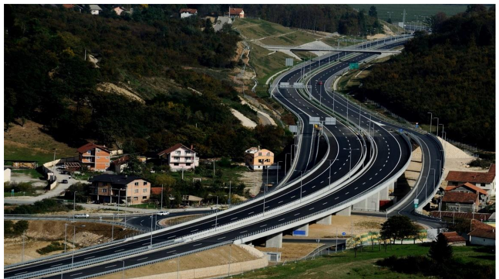
Newly built motorway on the Tarčin – Sarajevo – Zenica section on the Mediterranean Corridor (Vc) in Bosnia and Herzegovina.
